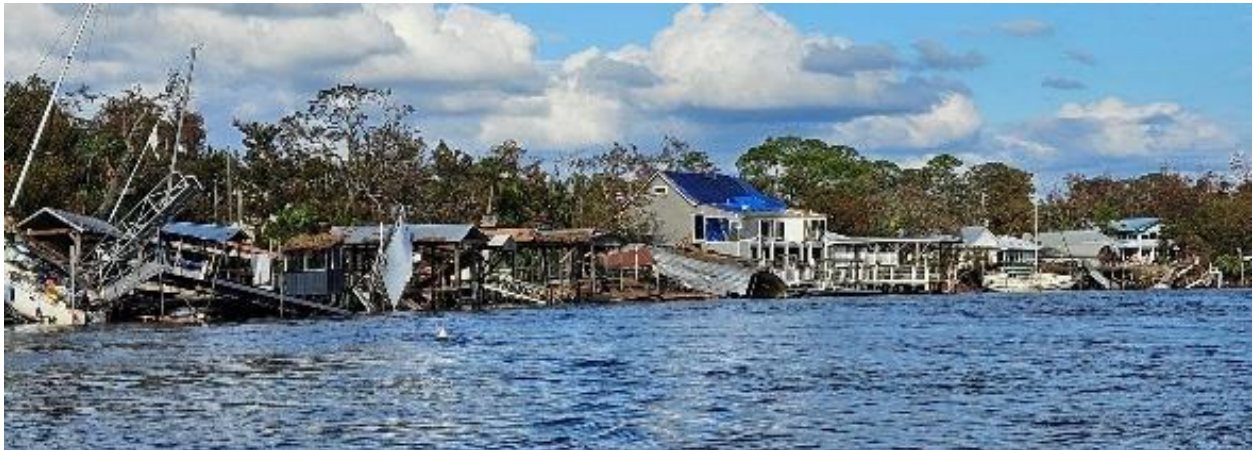
Photos illustrating the damage caused by Hurricane Helene in Taylor County.
